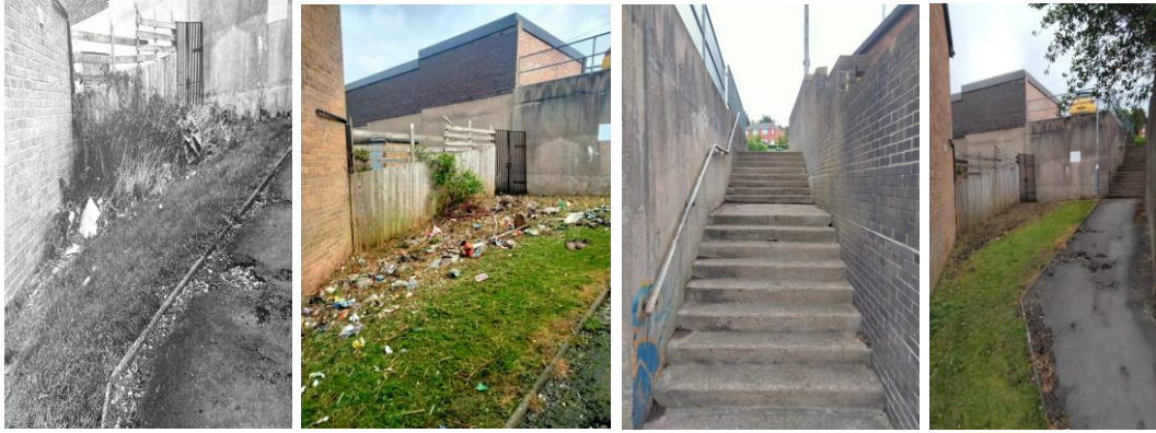
51. The team cleaned Amberley Road –‘Pigeon Poo bridge’ with great results.
